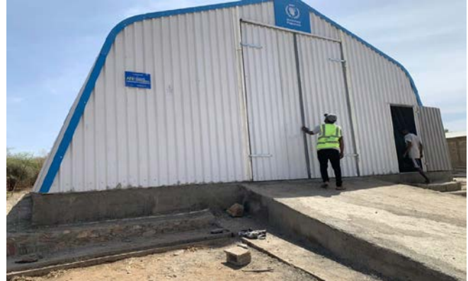
Flospan installation in Tigray operation
