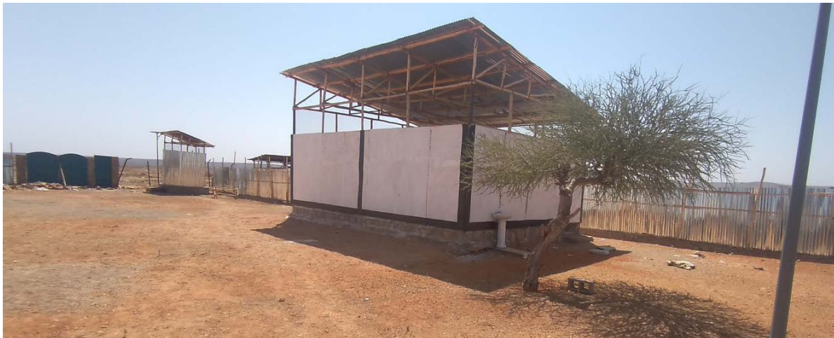
Covid-19 response Staff Station and toilet
