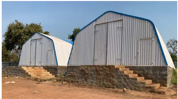
Flospan installation in Gambella operation
