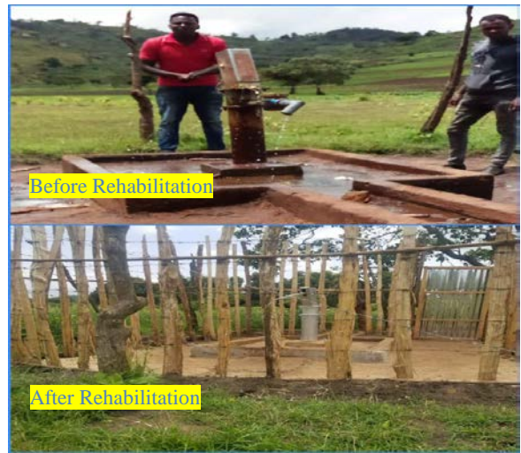
Shallow Well Rehabilitation of Medhiba
