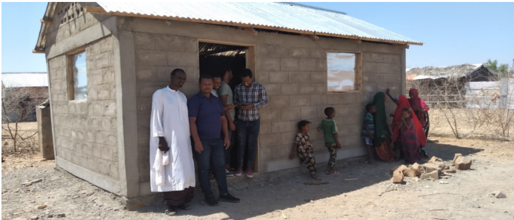
Improved Transitional Shelter Melikadida Operation
