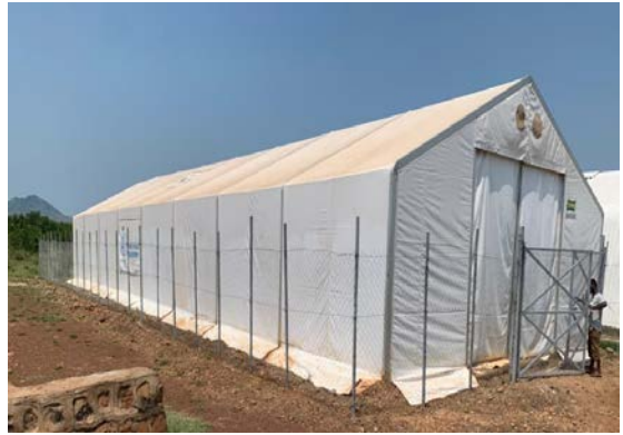
MSU Installation in Gambella Operation
