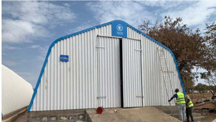
Flospan installation in Assosa operation
