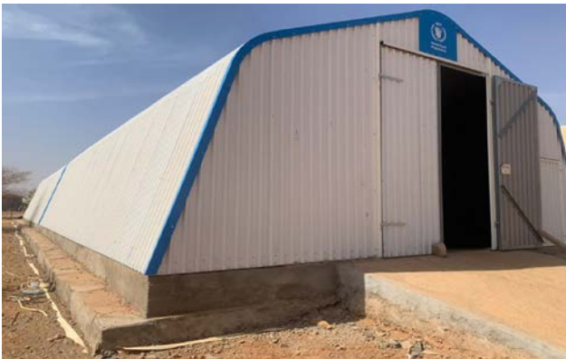
Flospan installation in Somalia operation
