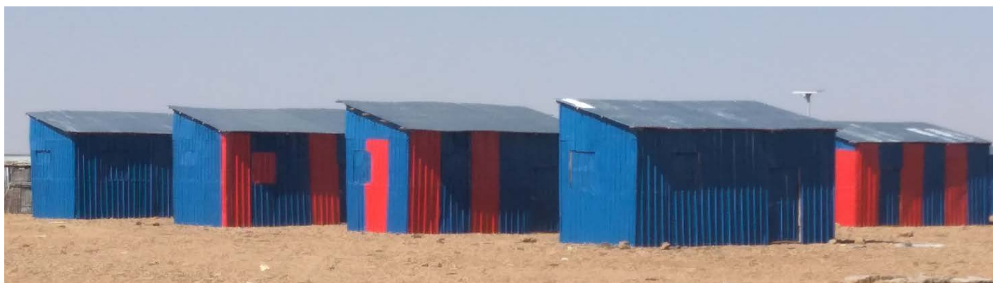
Standalone Emergency Shelter construction in Melkadida operation
