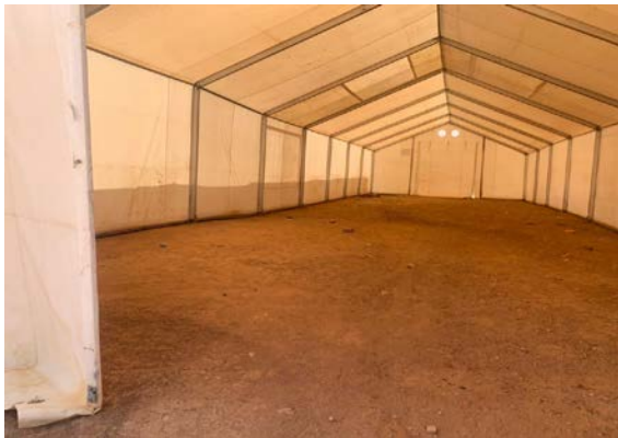
MSU Installation in Somalia operation
