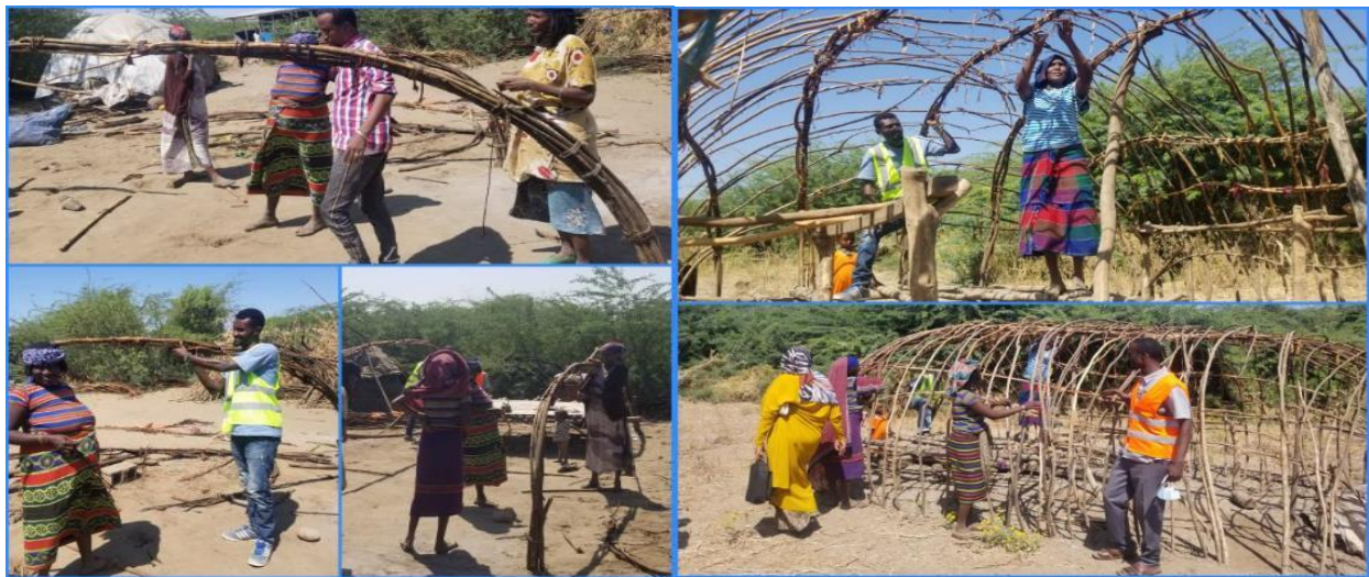
Figure-3: Photos taken during shelter construction demonstration.
